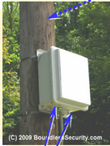
Exposed domes of two PTZ cameras provide wide views
