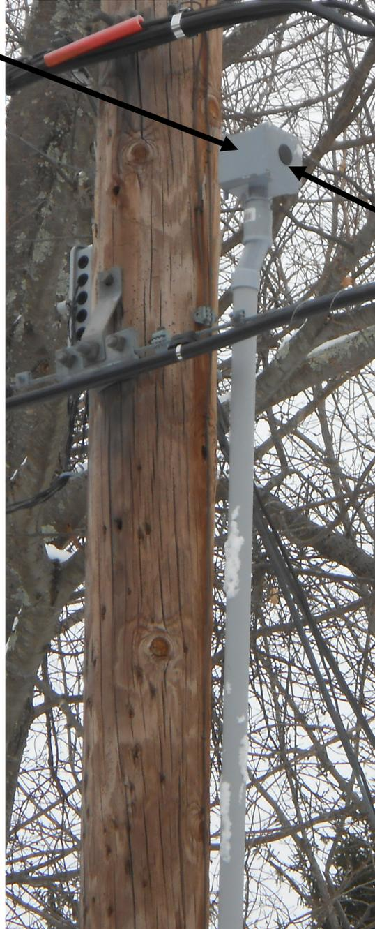
Mockup uses 1-1/4" PVC conduit (not incl) as example of rapid temporary installation from the ground. Antennas and ext. battery not shown.
